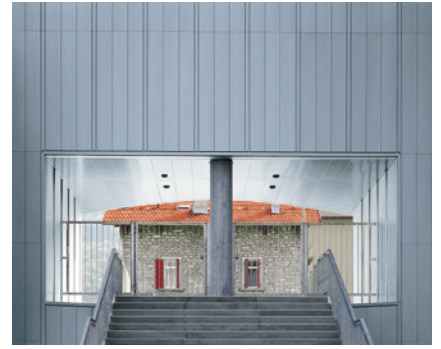
Telecom Giubiasco, Giubiasco, Schweiz
